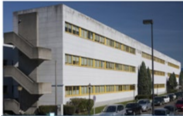
Civil Engineering School
